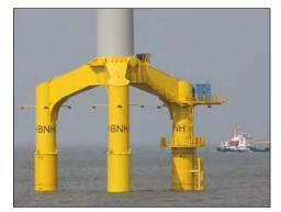
▲ Offshore wind turbine leveling: Enerpac's synchronous lifting system was the solution for leveling support cross pieces on 80 wind turbines.
